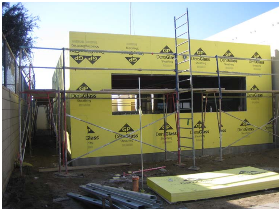
DensGlass Sheathing Added to the Exterior of the Addition
