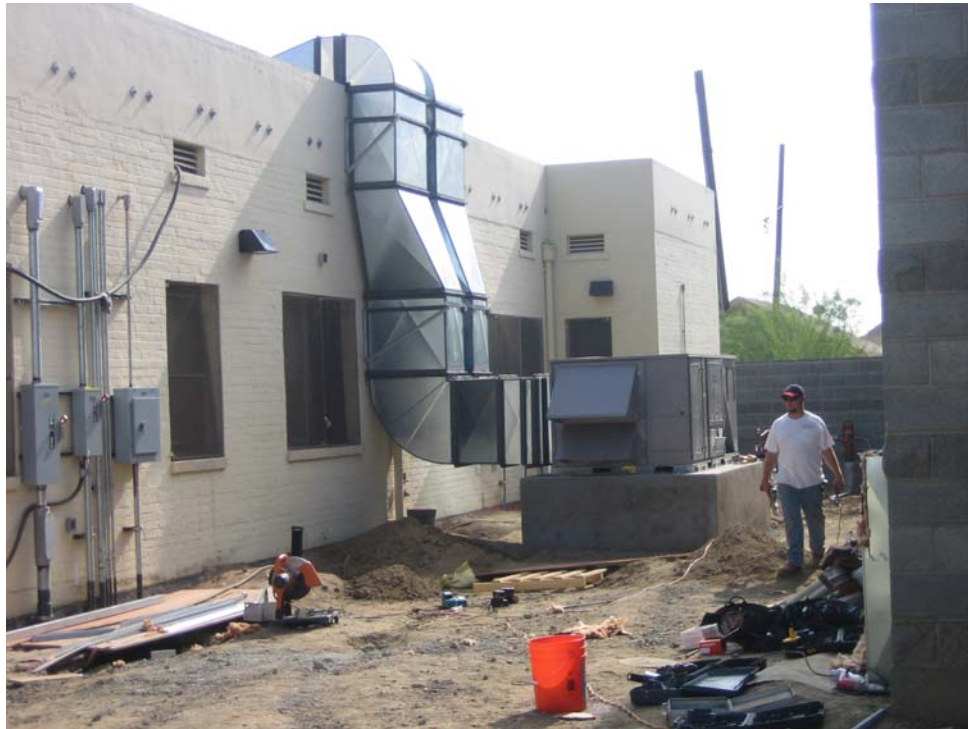
HVAC Unit Mounted On Pad
