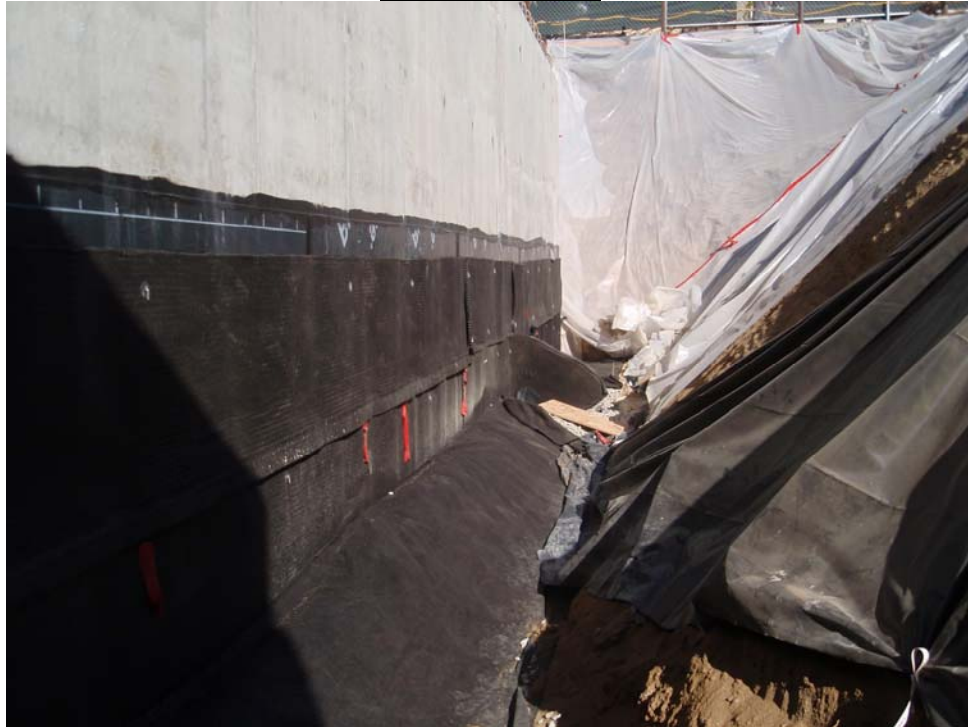
Installation of Wall Drainage System
