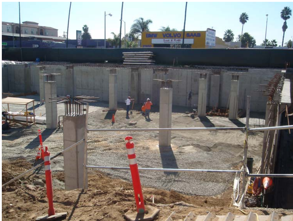
Preparation for Slab on Grade
