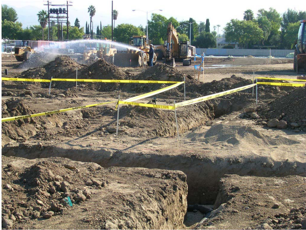
Excavation for Footings
