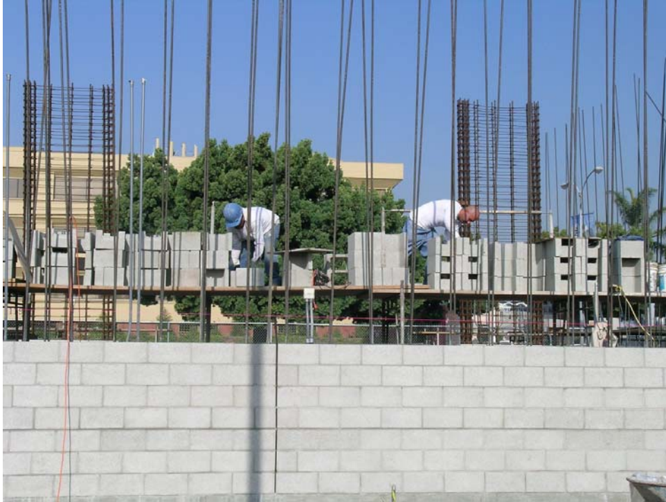
Second Masonry Lift
