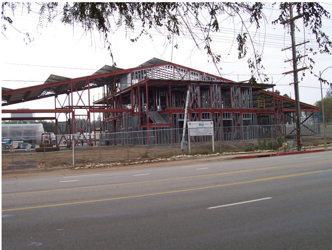
Fire Station Steel Framing
