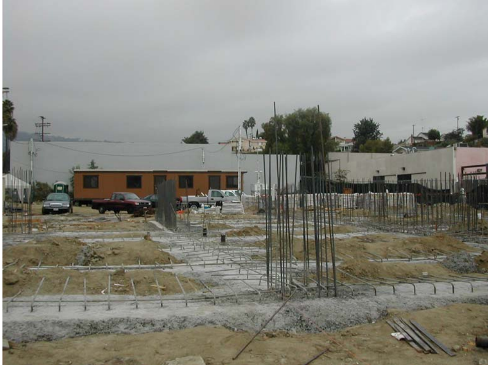
Grade Beam Installation
